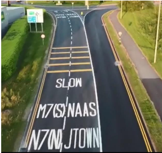
Restoration Improvement work - Naas
